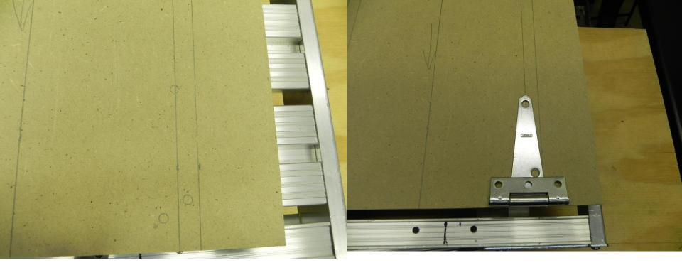
Place hinges on the backside of the seat and mark mounting locations. Drill holes and attach hinges to seats.
